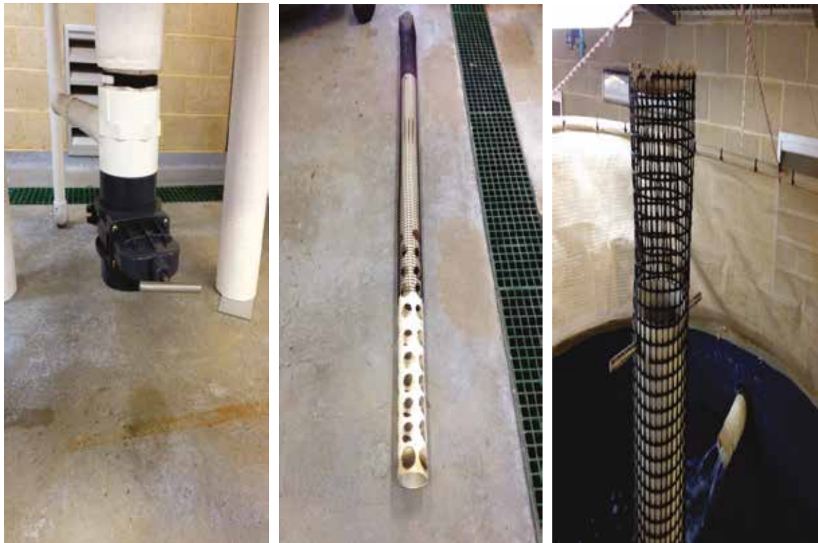
Figure 59. 2300 L tank components.
