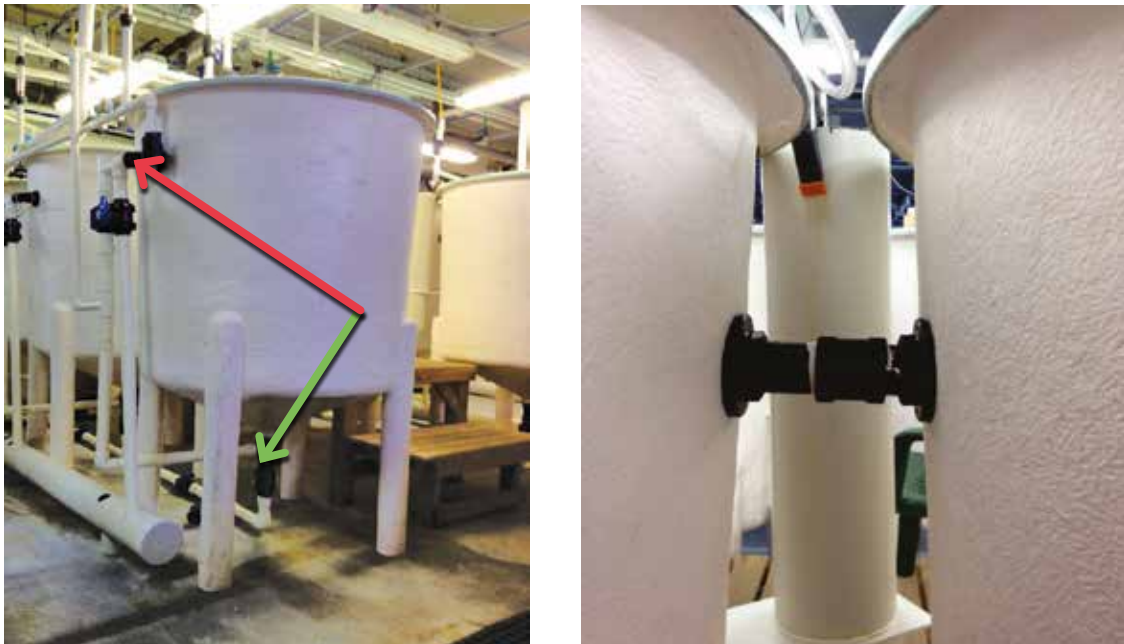
Figure 7. 1000 lt tank profile, green arrow indicating water inlet, red arrow indicating water outlet (left) two tanks connected with 40 mm tank fittings and joiner (right)
