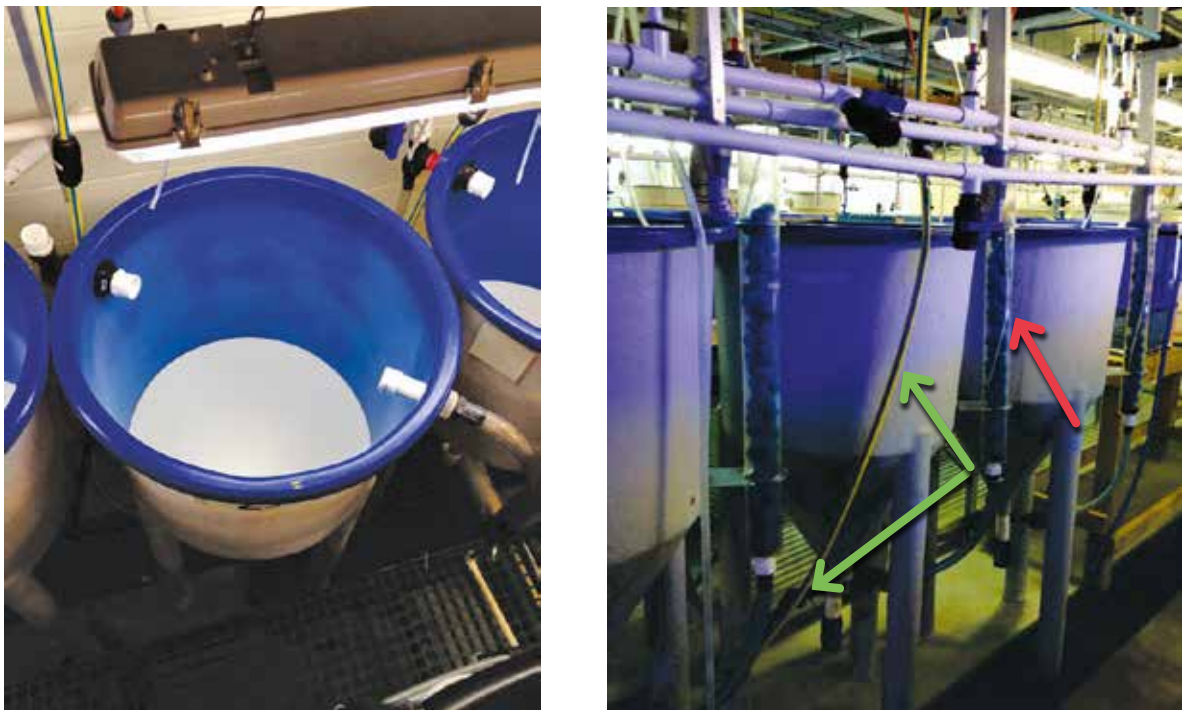
Figure 4. 270 lt tank profile and 32 mm outlet (left) seawater inlet options; red arrow indicating degassing column and green arrows indicating 20 mm flexible hose.
